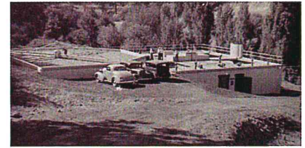
The Placerville Wastewater Treatment Plant at end of the project in 1938 (Courtesy of the El Dorado County Museum)
